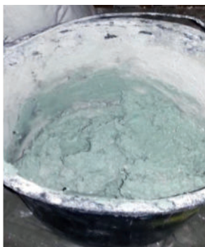
Mix GPG Marine to desired consistency
